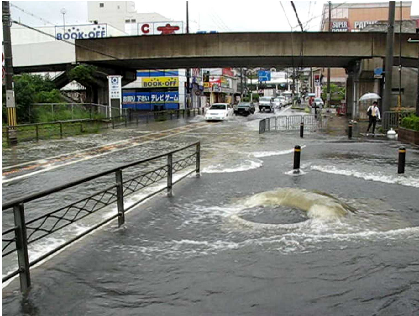
Overflow from a manhole at Rokujizo (六地藏)
