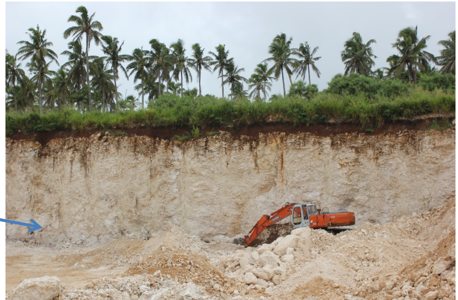
Picture of the exposed limestone aquifer in a quarry 5 km south-east of the Matakī'eua well field
