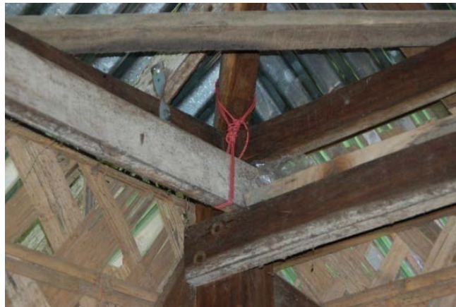
Linking the joint with bolt
