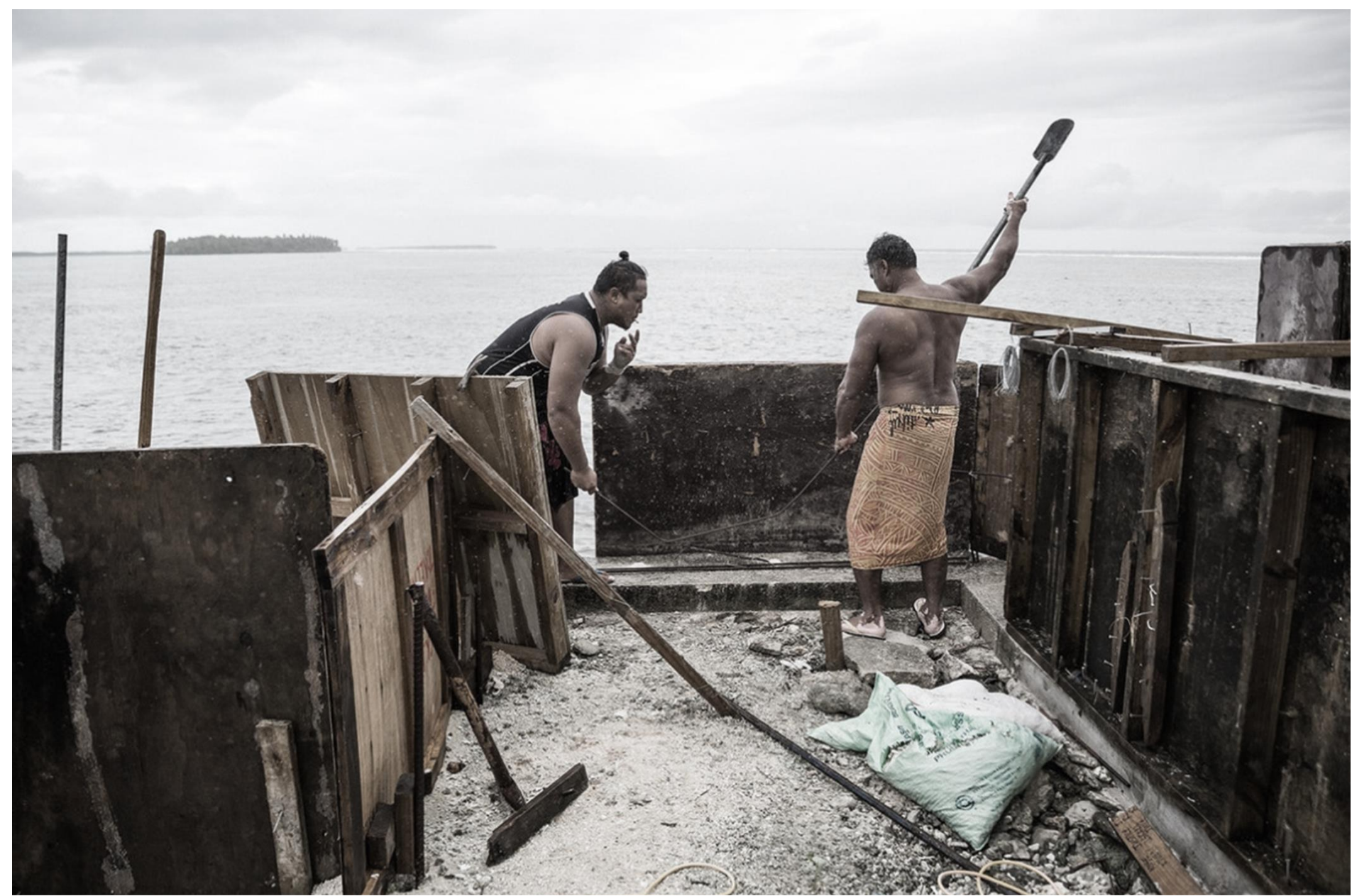
A FATHER AND SON BUILDING A 5 TO 7 METER HIGH SEA WALL IN FRONT OF THEIR HOUSE IN AN ATTEMPT TO FIGHT THE RISING SEA LEVELS.
